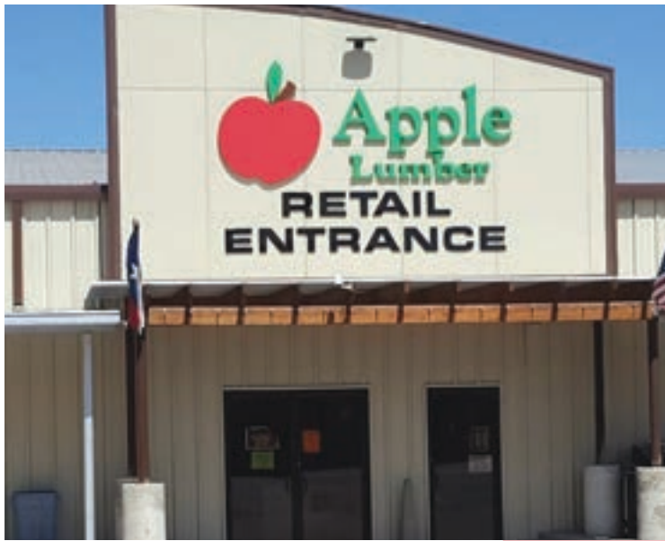
This is the entrance to the retail store in Yorktown.
